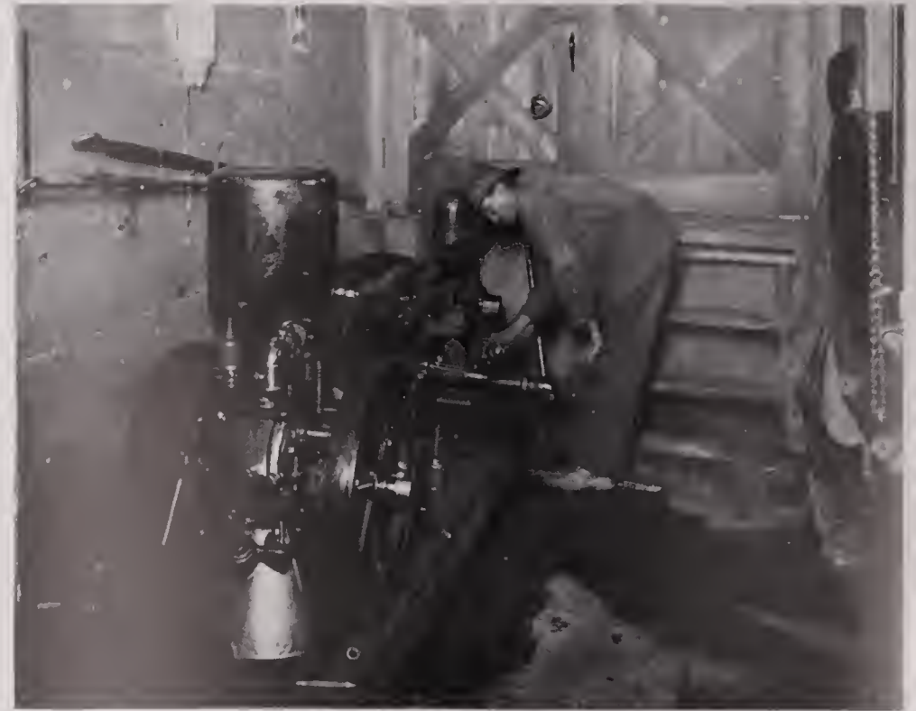
THIS PUMP SUPPLIES PURE WATER FROM DEEP WELL
